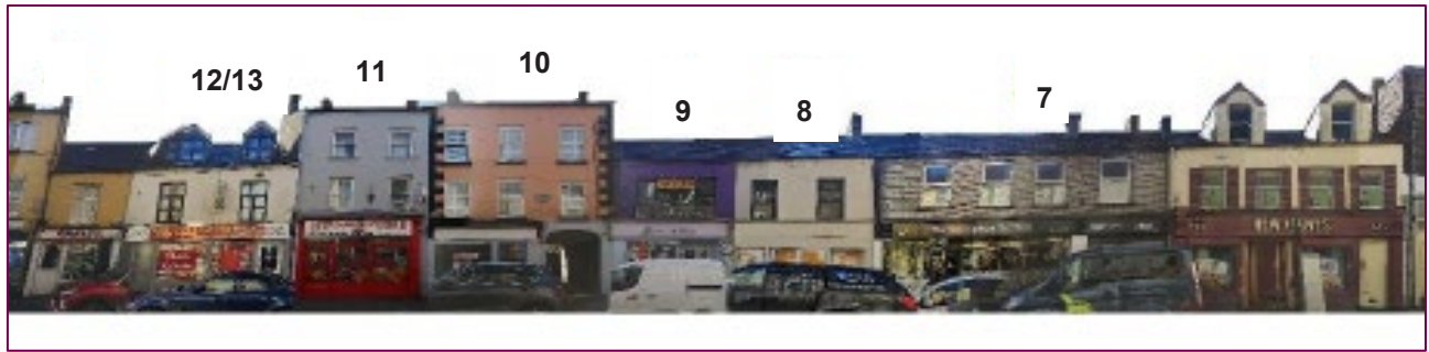
Figure 4.3:: Buildings Proposed for Demolition along Dublin Street
