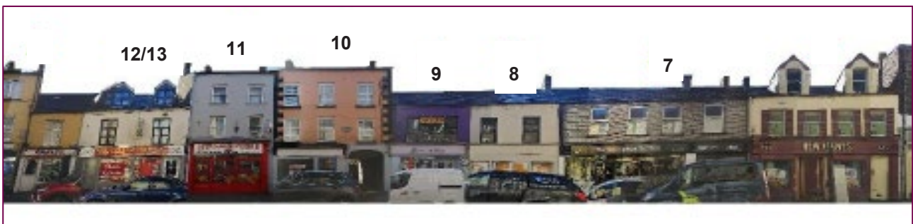
Figure 2.7: Buildings Proposed for Demolition along Dublin Street
