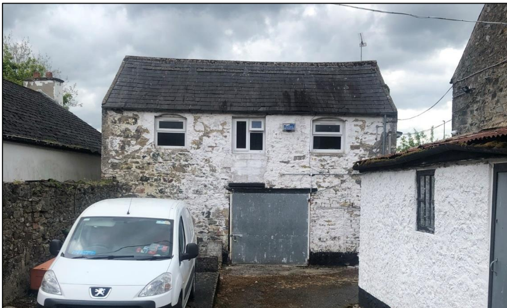
Figure 15.9.8.3.4: Outbuilding for demolition to rear of Sherry’s Public House
