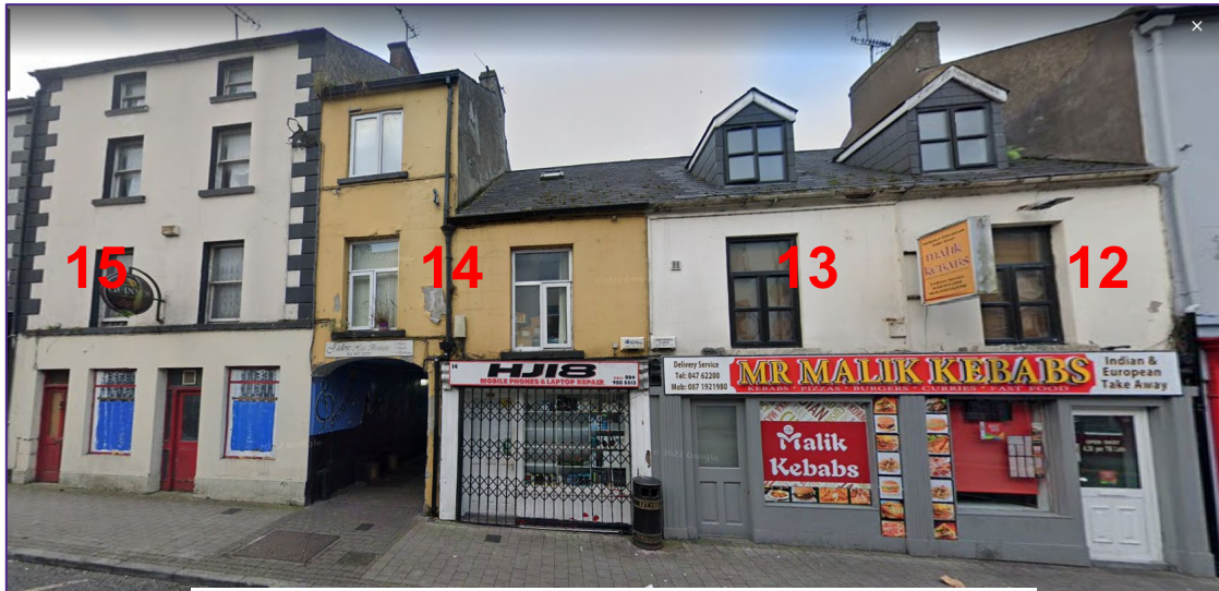
Figure 2.25: Frontage Buildings at 12-15 Dublin Street
